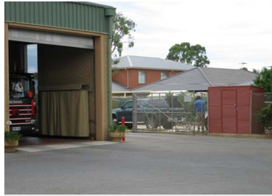
New station delivery shed at Brooklyn Park Fire Station
