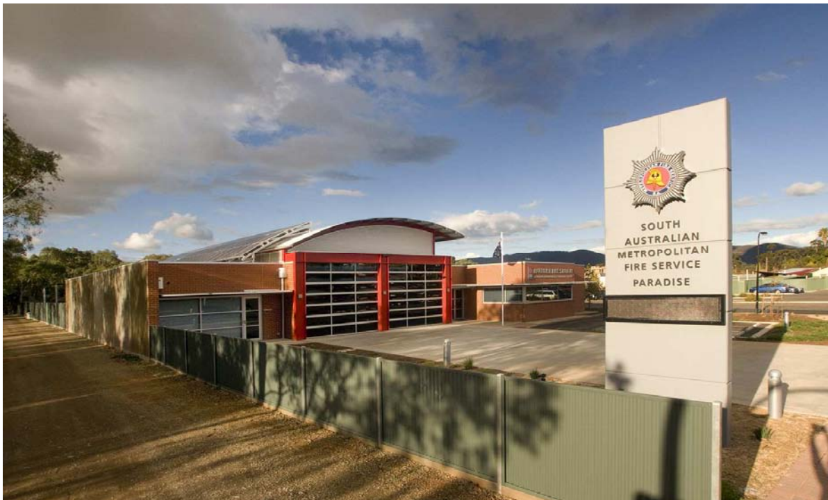
View of Paradise Station showing contoured solar panels
