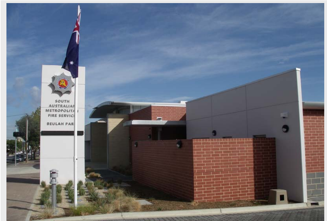
The new Beulah Park Station
