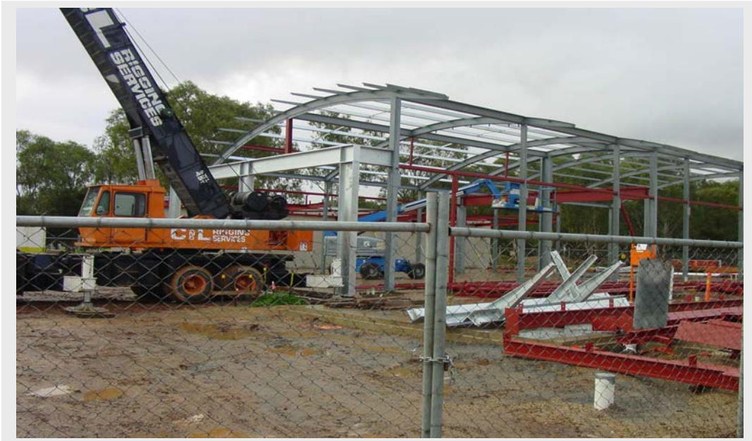
Work underway at the new Paradise Station
