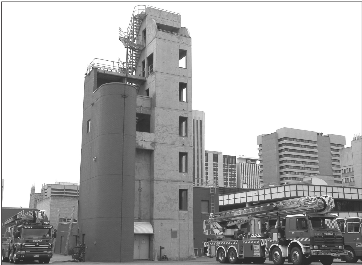
Breathing Apparatus and Training Complex, Adelaide Fire Station
