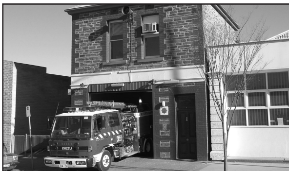
Heritage listed Kapunda Fire Station
