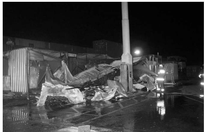
Container Fire, Outer Harbour On 5 December 2003 over $1 million fire damage was caused in the crane electronics maintenance section at Outer Harbour. The fire was accidental, caused by portable radio chargers overheating.
