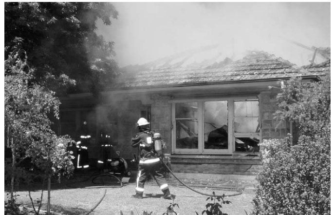
House Fire, Firlie An electrical fault in the ceiling wiring caused $500,000 damage to this house on 27 February 2004.
