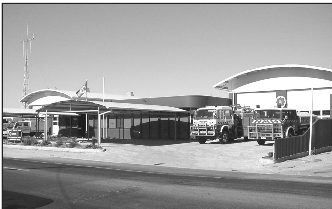
The new Renmark Emergency Services Centre
