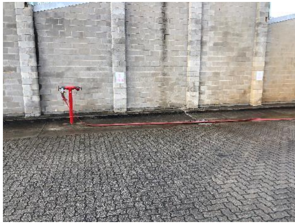
Photo 21 Wash down area facing east from rear of MFS building
