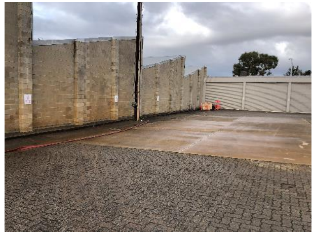
Photo 22 Wash down area facing south-east from rear of MFS building
