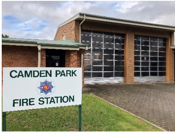
Photo 19 View of the front entrance facing east from Morphett Rd
