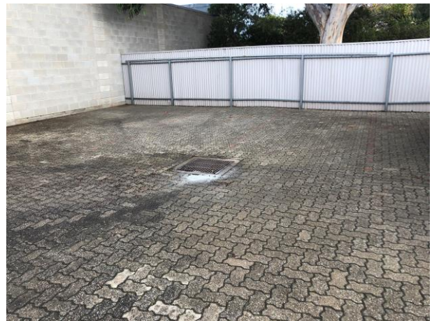
Photo 24 Drain in south-west corner of site
