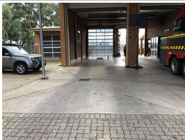
Photo 2 Truck wash bay from rear, facing north
