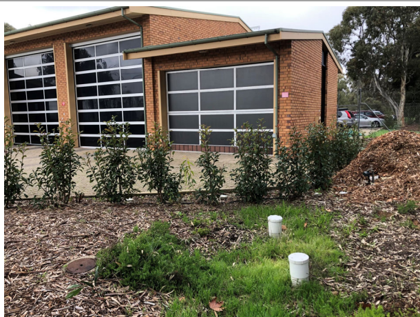
Photo 1 View of station from NW corner of building from Grand Junction Rd, facing south. Irrigation visible
