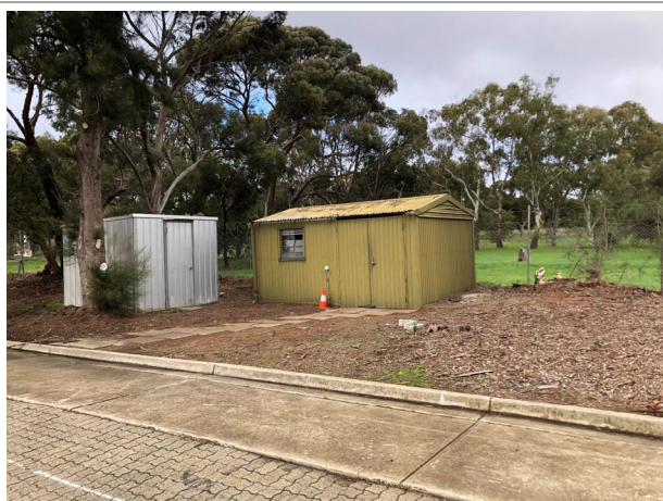
Photo 3 Storage sheds, facing south-east
