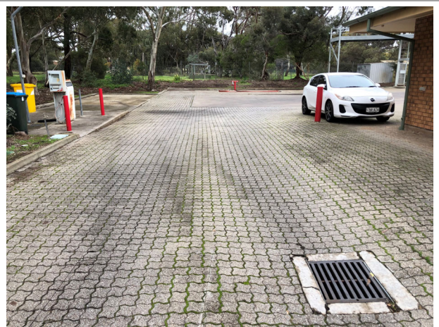
Photo 10 View of driveway with stormwater pit/ drain, decommissioned fuel pump and the former dam, facing south
