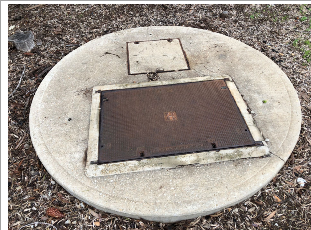
Photo 11 View of decommissioned 15,000 L diesel underground storage tank, facing east
