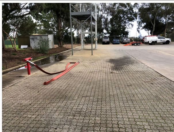
Photo 4 View of training area and hydrant, facing west
