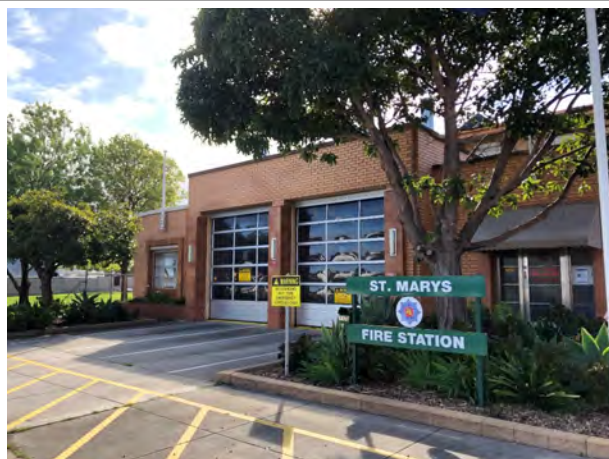
Photo 1 Front entrance of station facing west on South Road
