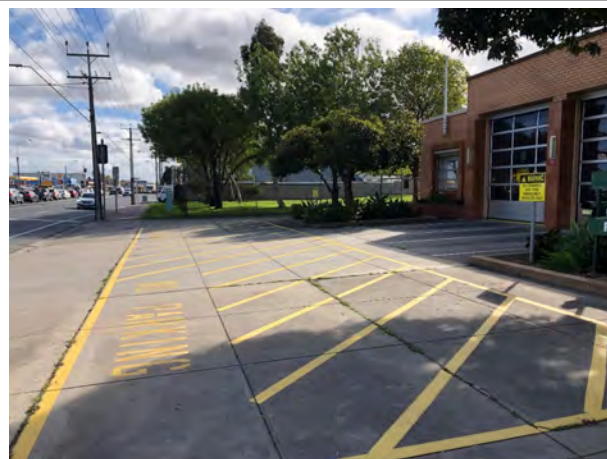
Photo 2 Front apron on South Road in front of the north-western training area, facing north
