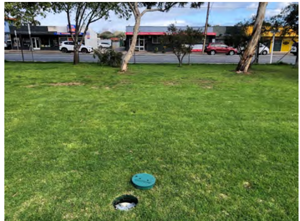
Photo 16 Groundwater monitoring well 6628-31030 in north-west training area facing west
