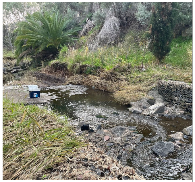
Photograph L: Christie Creek near SW13 showing rock gabions, some bank erosion, grasses and weeds.
