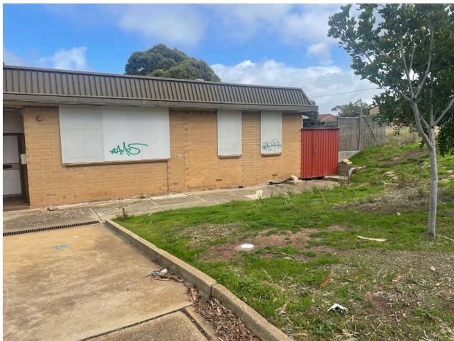
Photograph E: North-eastern corner of the site, facing north-west (post closure).
