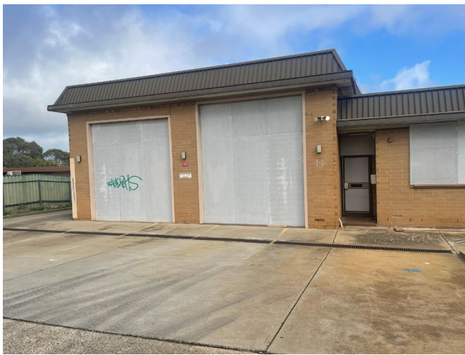
Photograph C: South-eastern corner of the site, facing south-west (post closure). Driveway and drain located to the east of the building.
