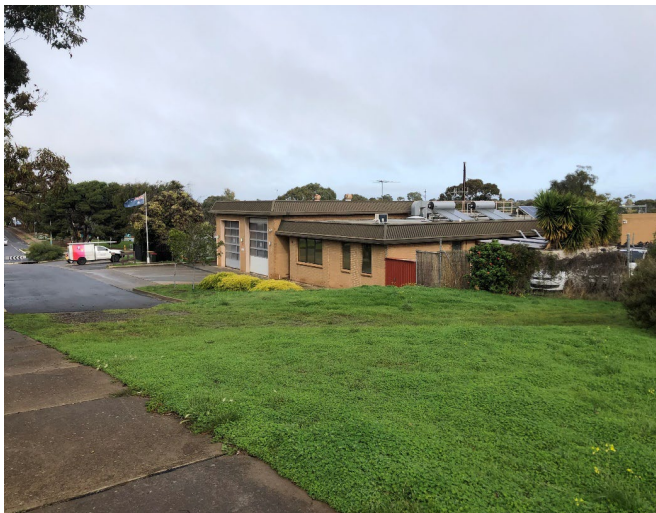
Photograph A: North-eastern corner of the fire station, facing south-west (prior to closure). Grassed area outside of the fence.
