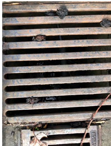
Photo 10 Close up of stormwater drain
