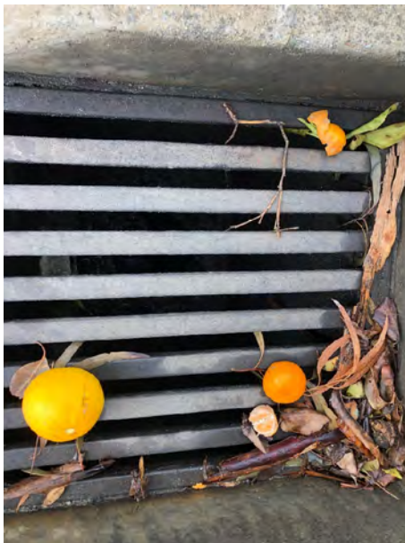
Photo 9 Close up of stormwater drain
